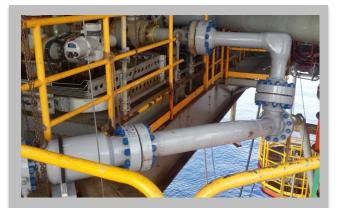
Flexi-Coil® Velocity string can be deployed through multiple surface pipework bends allowing access to the production riser without direct vertical access and hung off in a surface hanger.
